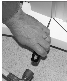
Tap in screwdriver blade at base
